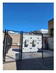
Above, for comparison and reference, is a photo of the Telluride High School microgrid BESS package with concrete pad and safety/security fence. This system is about half the size of the system being considered for the Ophir Microgrid.
