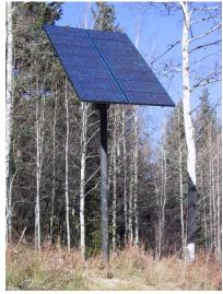
An example of a pole mounted solar array that is installed high enough to handle the anticipated snow accumulation.
