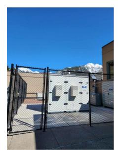
Above...Telluride High School BESS package with concrete pad and safety/security fence.
