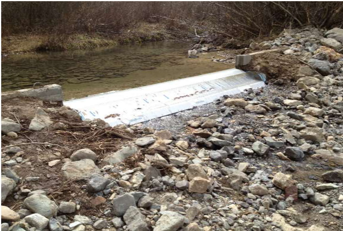
Figure 5: Town of Ophir's raw water intake off Waterfall Creek
